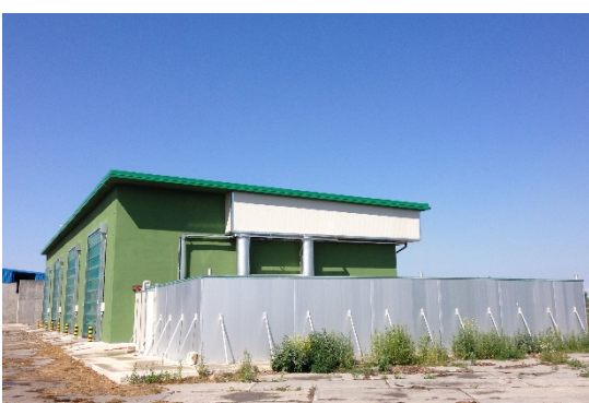
(4) BIOFILTER TO TREAT PROCESS AIR EFFLUENTS
